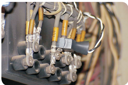
Fig. 4 and 5: CT donut connections to the secondaries of the protection CTs.
