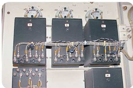
Fig. 4 and 5: CT donut connections to the secondaries of the protection CTs.
