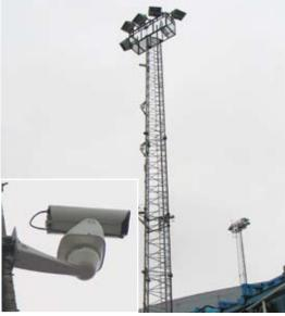
One of the FLIR Systems SR-100 thermal imaging cameras installed
